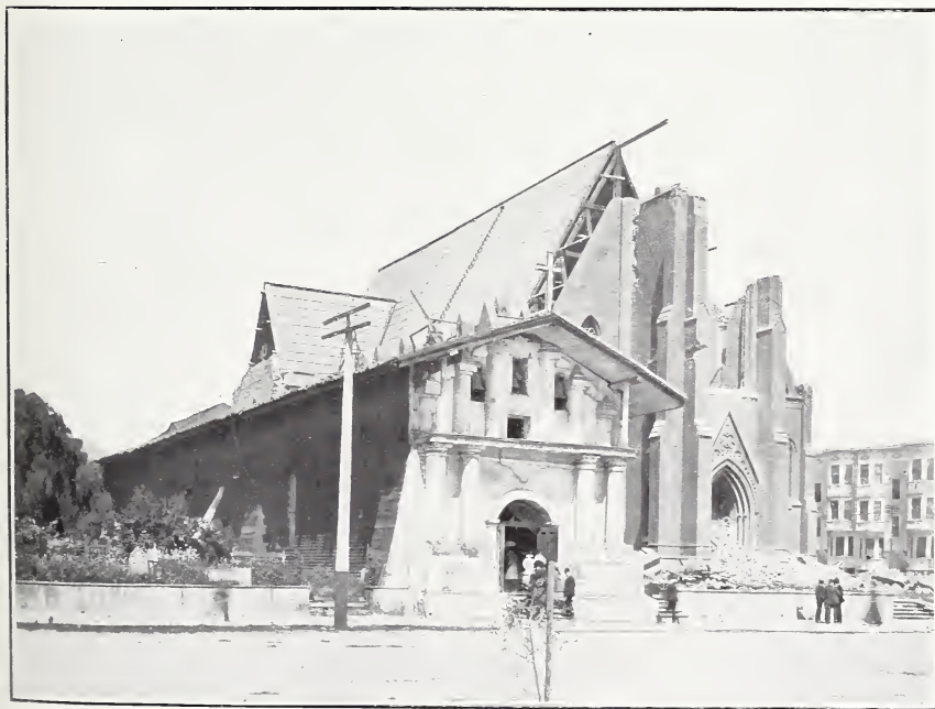
B. EFFECT OF EARTHQUAKE ON ADJACENT BUILDINGS OF DISSIMILAR TYPE AND CONSTRUCTION.
